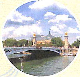
"Pont Alexandre III"
